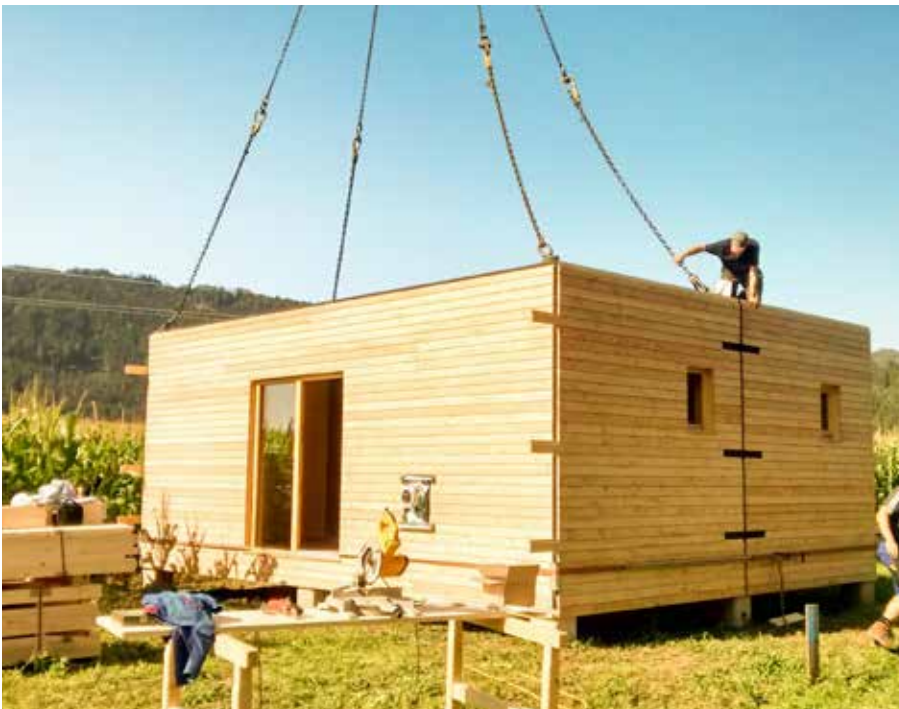
The Holz100 Mobile Home is constructed so that they can also be stacked.
